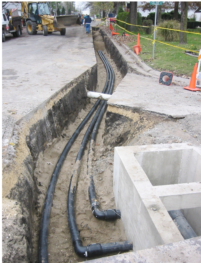
More trenches like this one will be installed in selected areas of northern Hartford. These trenches hold piping that carry vapors removed by the extraction wells to the refinery property where it is then burned in thermal oxidizers.
