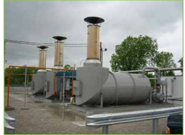
Multiple thermal accelerators treating free product vapors from a pipeline break.
