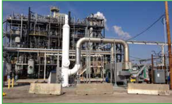
Recuperative Thermal with HCL scrubber
